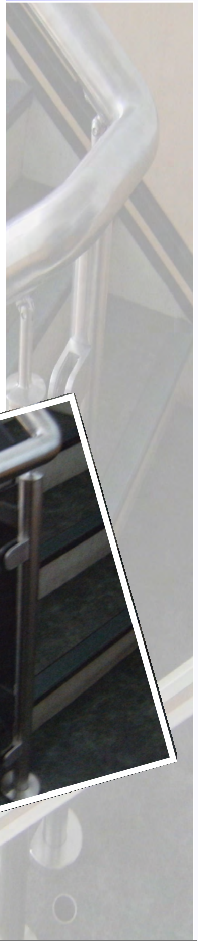
Trade Mouldings—Stainless Steel Balustrade to stairs with tinted glass
